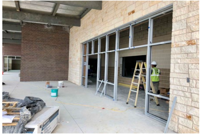
Exterior: Area 4, rear entry storefronts being installed.
