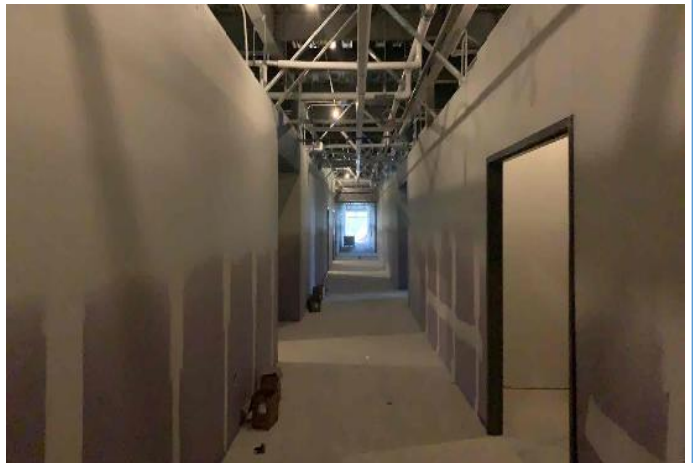
Interior: 1st floor walls texture and paint has begun.
