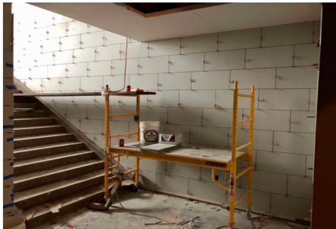
Interior: Wall tile in stairwells has begun.
