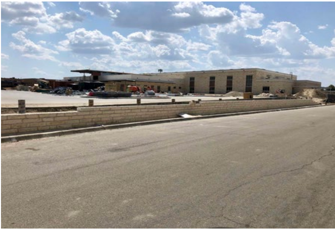
Site: Retaining wall on Lydia Drive.
